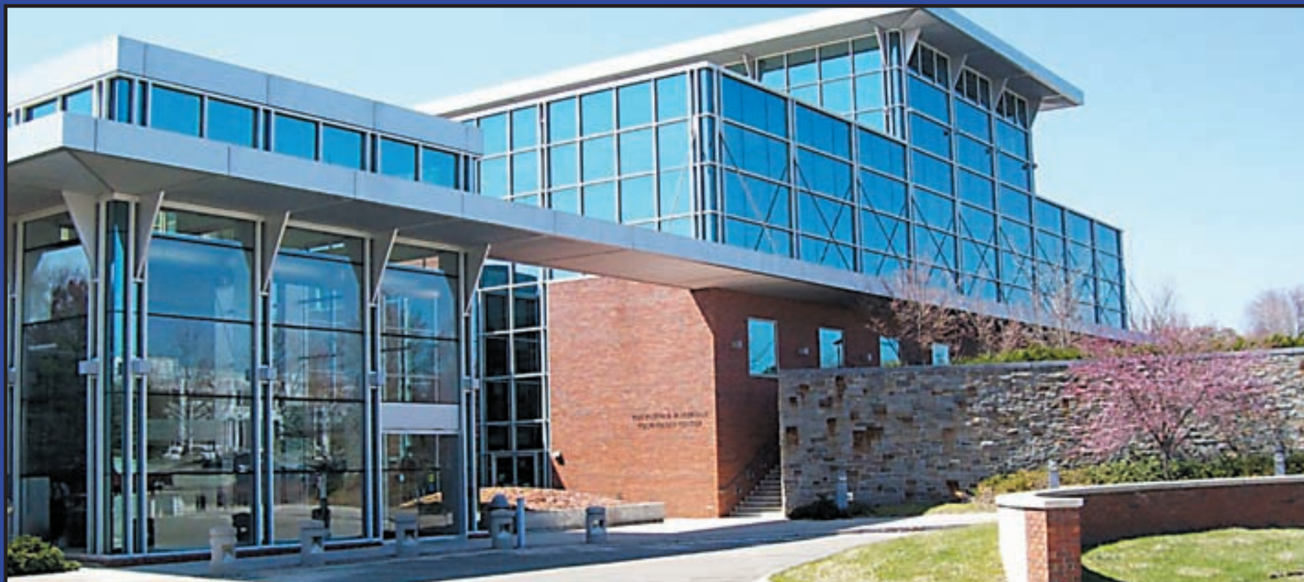
Sentinel Data Center - Trumbull, CT
