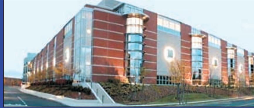
Sentinel Data Center - Needham, MA
