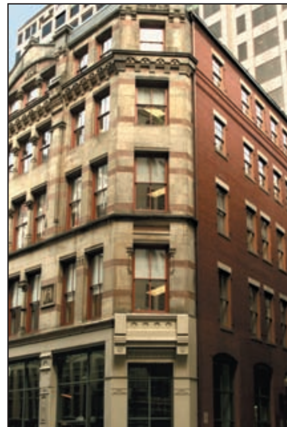
101 Arch St. Renovation
